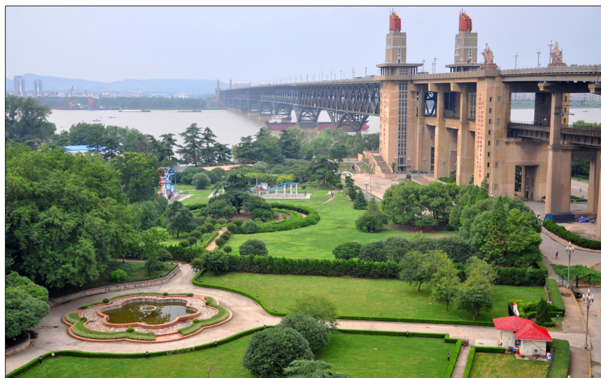
Photo Courtesy of Adobe Stock - The Nanjing Yangtze River Bridge
