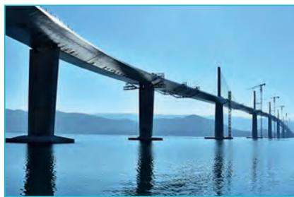
**Cortec's MCI® 2018 was specified on Peljesac bridge project as a silane-based impregnation with a migrating inhibitor property to protect against the harmful effects of corrosion**
